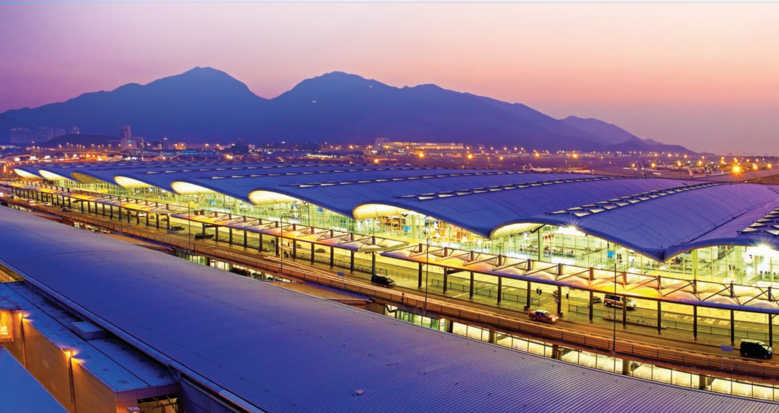
Hong Kong international airport
